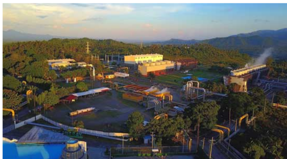
Makban Geothermal Power Plant
